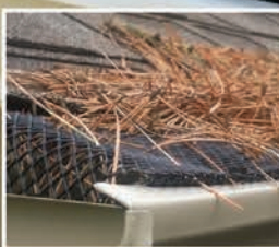
Filter Systems Still stacked up with water- blocking debris.
