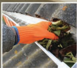
Unprotected Gutters Clogged with all kinds of gunk.
